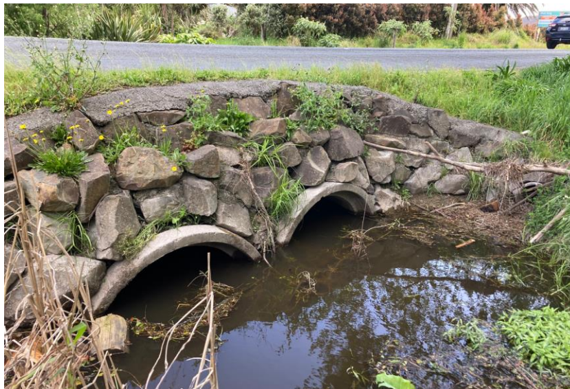
Figure 7-4: Twin 1.2m diameter culverts under Mangawhai Heads Road (West).
