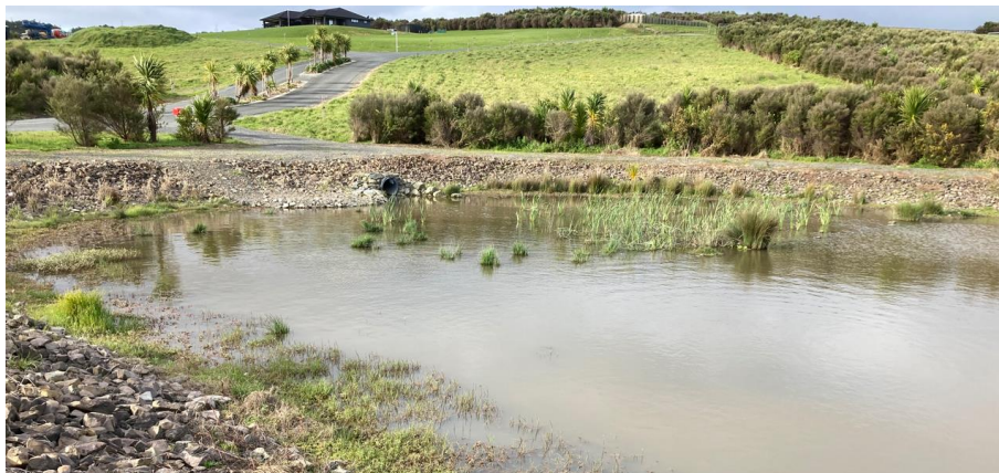
Figure 7-9: Stormwater pond on Lot 8 DP 533510 within the PPC Area
