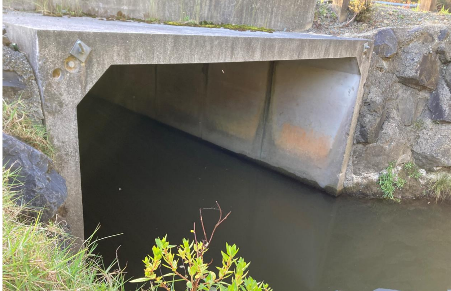
Figure 7-5: Box/bridge culvert under Cove Road
